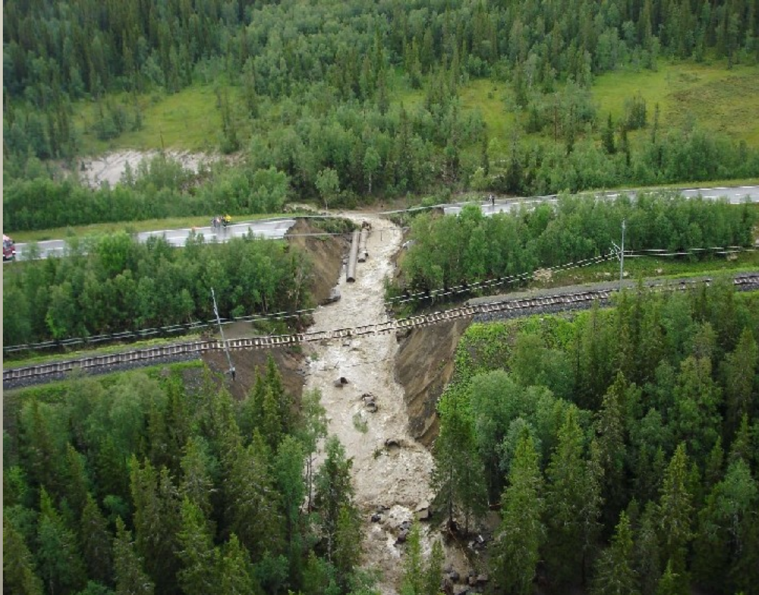
Landslide at Enafors, Jämtland, 2006
