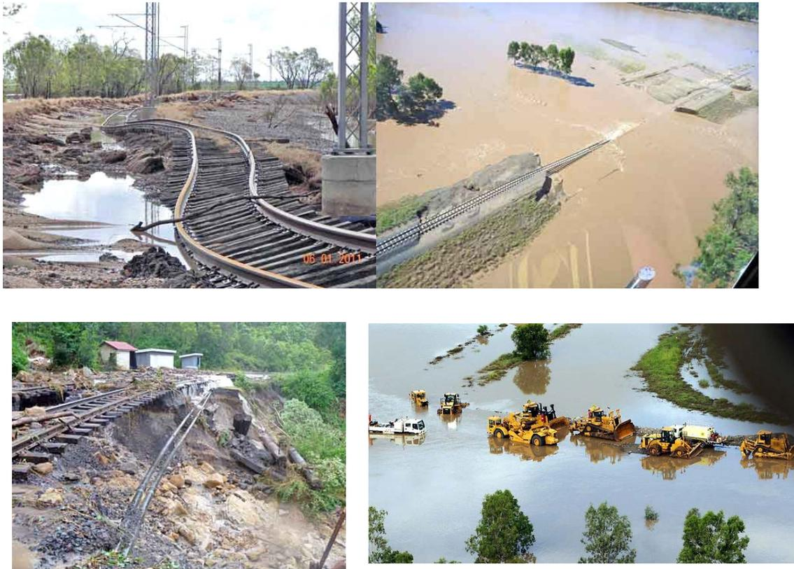
Figure 13: Images of destruction to Queensland rail lines – 2011 floods (Top left: Queensland floods, 2011a, Top right: Queensland floods, 2011b, Bottom left: Toowoomba Range damage, 2011, Bottom right: Mechielsen L. 2011)
