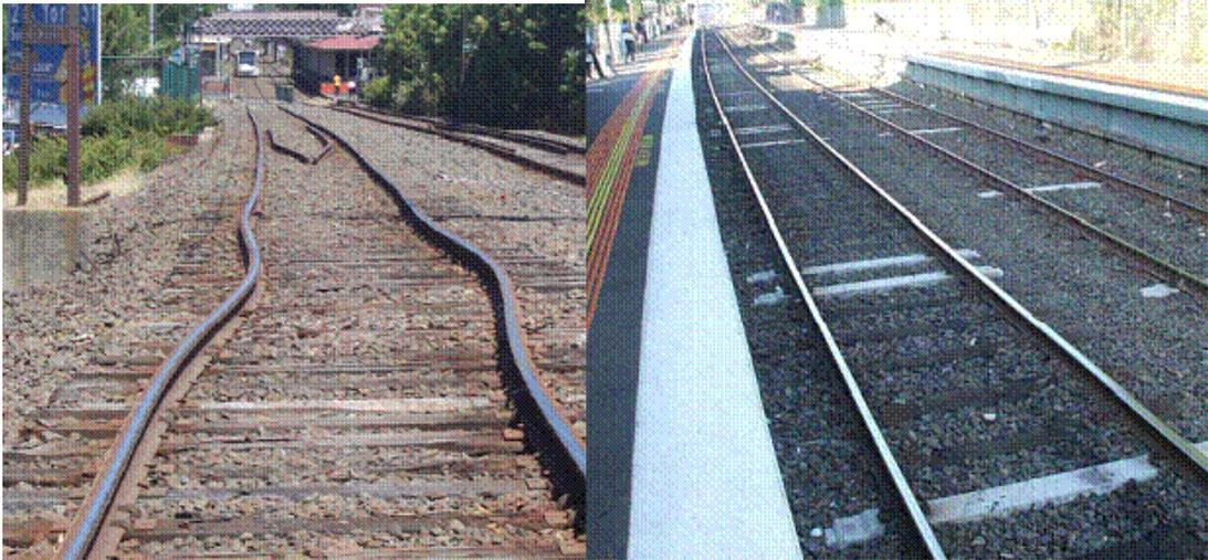
Figure 5: Rail buckling and replacing old timber sleepers with concrete sleepers (Metcalfe et al. 2009)
